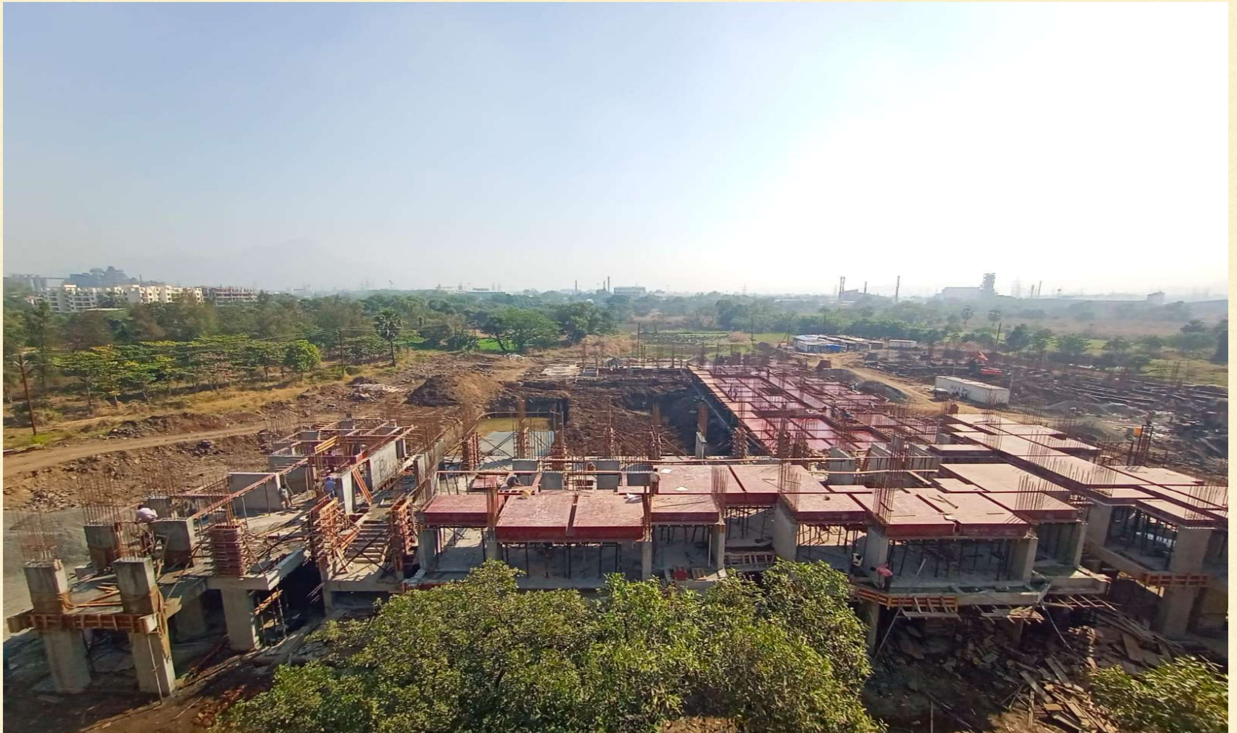
Slab work in progress for R & S wing, Plinth work in progress for T wing
