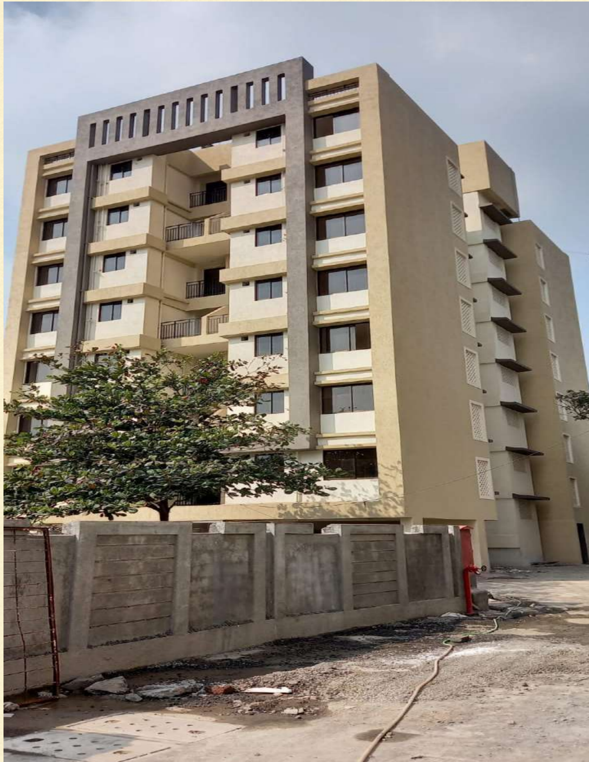
Flooring & Tiling, Doors & Windows completed
