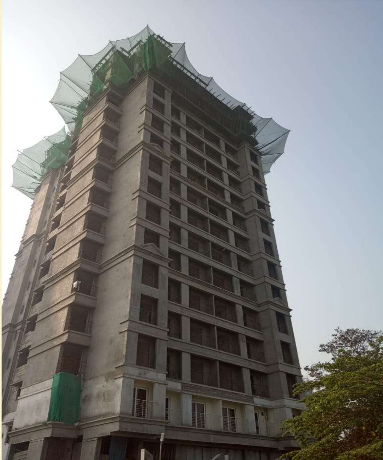
Flooring, tiling, kitchen works in progress
