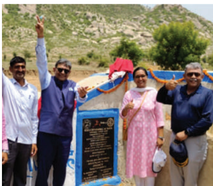
Contributed towards the construction of a check dam
