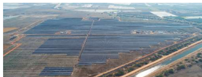
30 MW capacity solar power plant located in Raichur district of Karnataka state under group captive model
