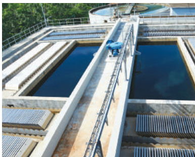
Ultra High Rate Solids Contact Clarifier (UHRSCC) Flow rate: 1500 m 3 /h
