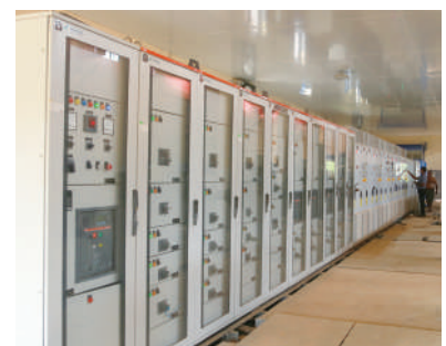
Water Treatment Plant (WTP) pump house main MCC panel (APFC, VFD, AHF)
