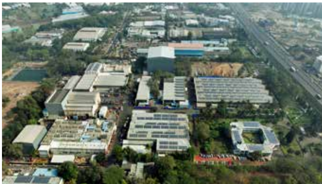
CG's Switchgear Manufacturing Unit in Nashik, Maharashtra
