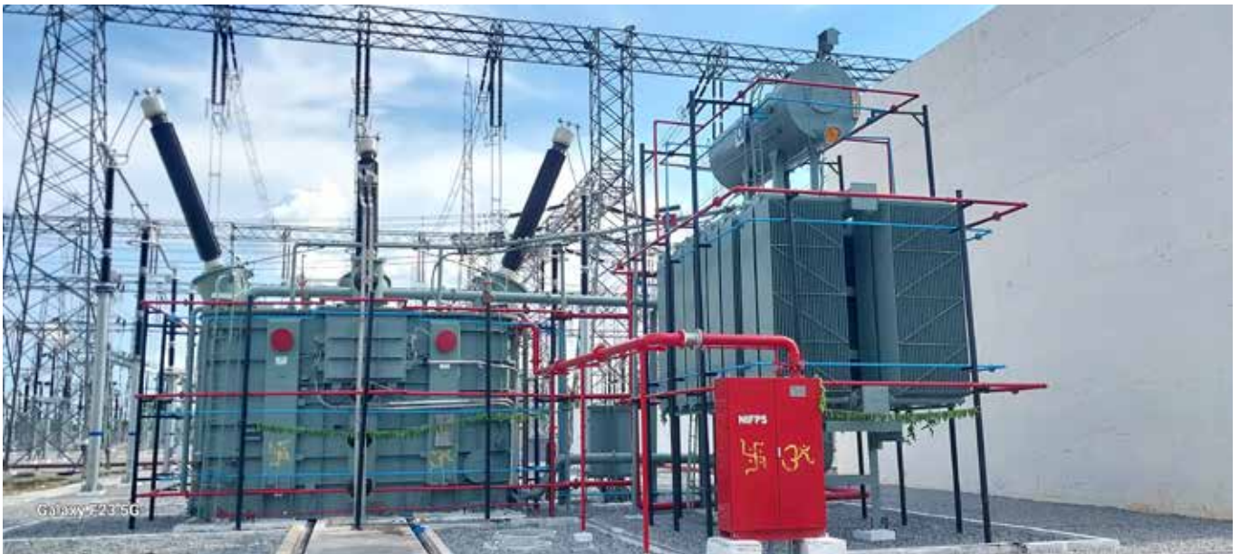
125MVA r 400kV 3-Ph Reactor Supplied by CG for TS Transco Project
