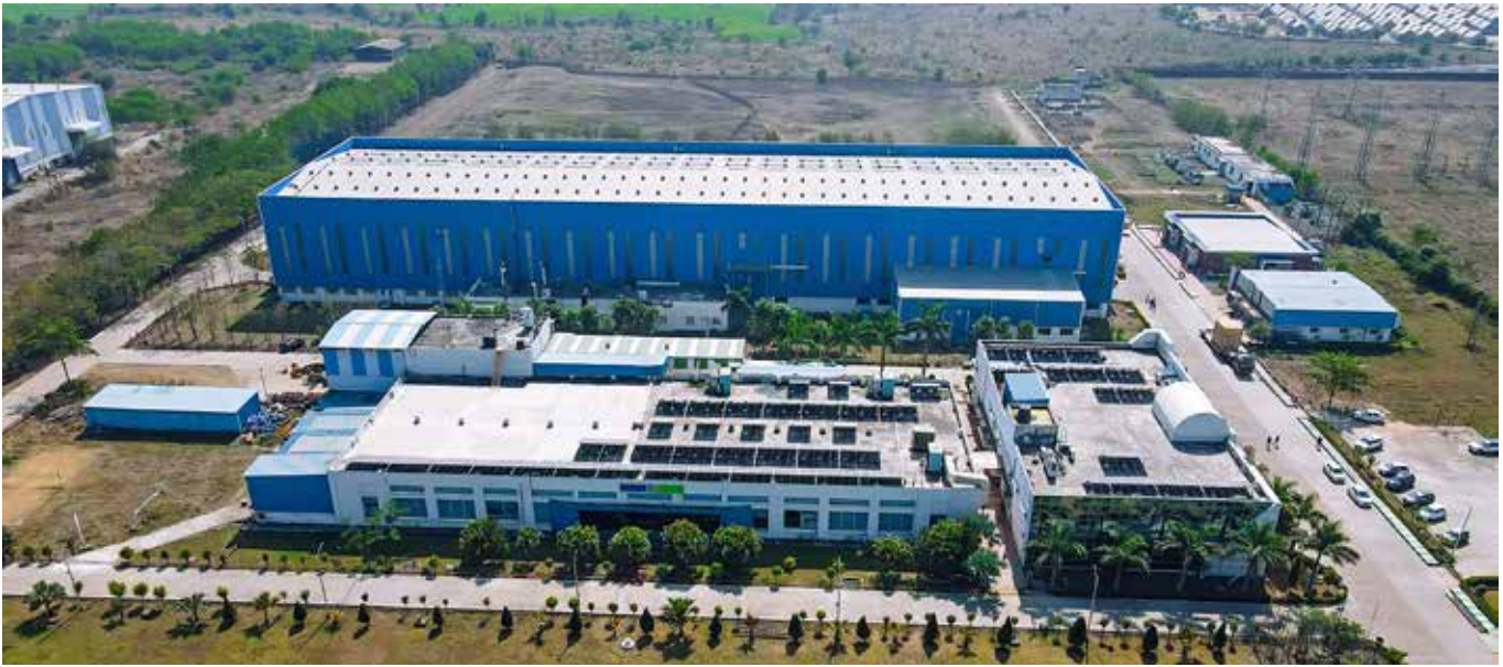
CG's Motors and Drives Manufacturing Unit in Bhopal, Madhya Pradesh
