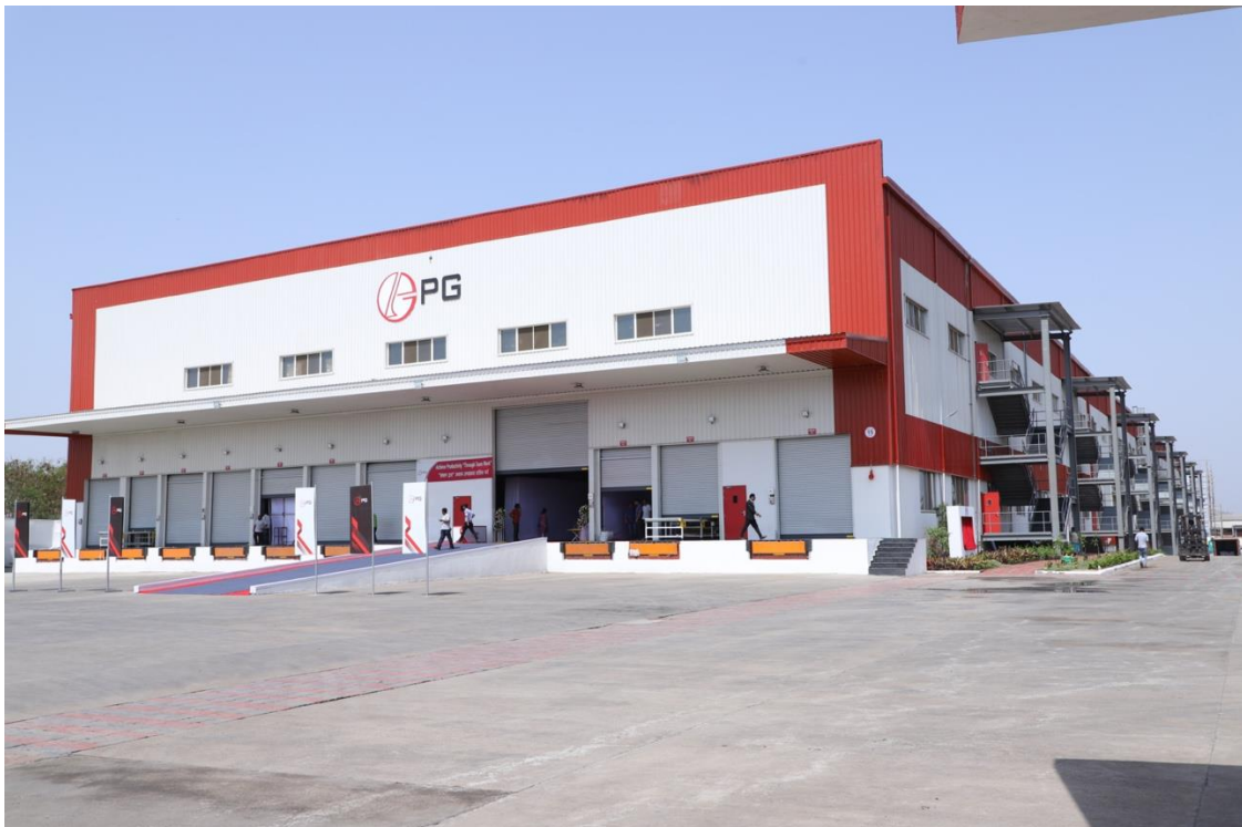
Image: Flagship Integrated AC Manufacturing Facility
