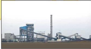
CAPTIVE POWER PLANTS (143 MW, MULTI-FUEL)
