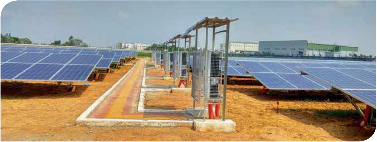
Thermax commissioned a 1.285 MW ground mounted solar photovoltaic system for a leading consumer brand's manufacturing facility at Sri City, Andhra Pradesh. The system is integrated with diesel generator sets to minimise the customer's fuel consumption and dependence on grid power.
