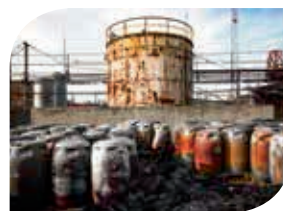
Hazardous Waste Treatment
