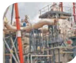
Tank Farm Heating
