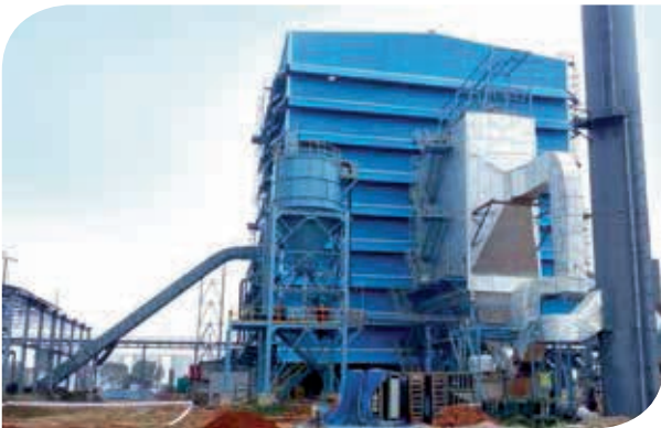
The Power EPC division commissioned its 100 th power plant during the year.
