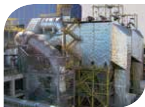
Air Pollution Control
