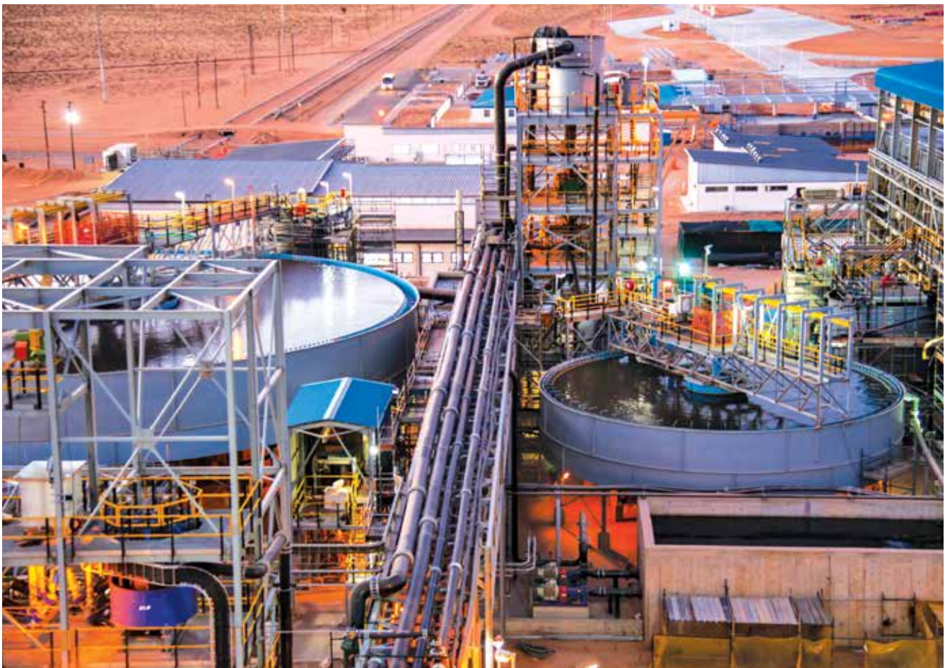
Gamsberg Wet Area (Flotation, Thickener)
