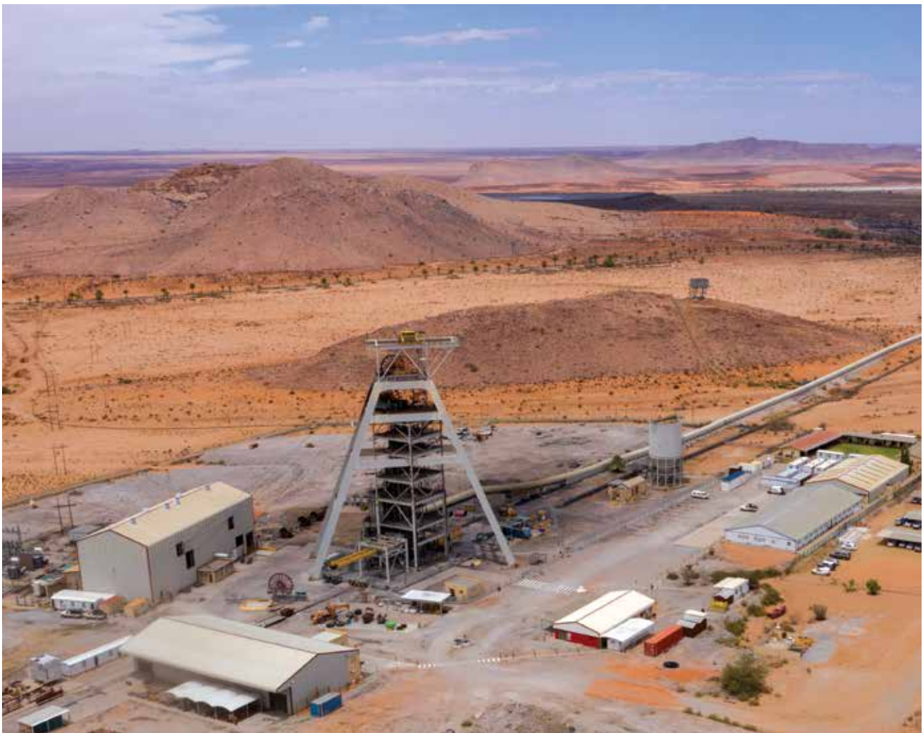
Deeps Shaft at Black Mountain Mine
