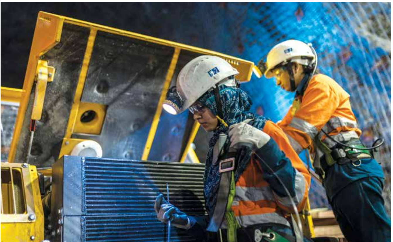
Women conducting maintenance work in the Rajpura Dariba Mine
