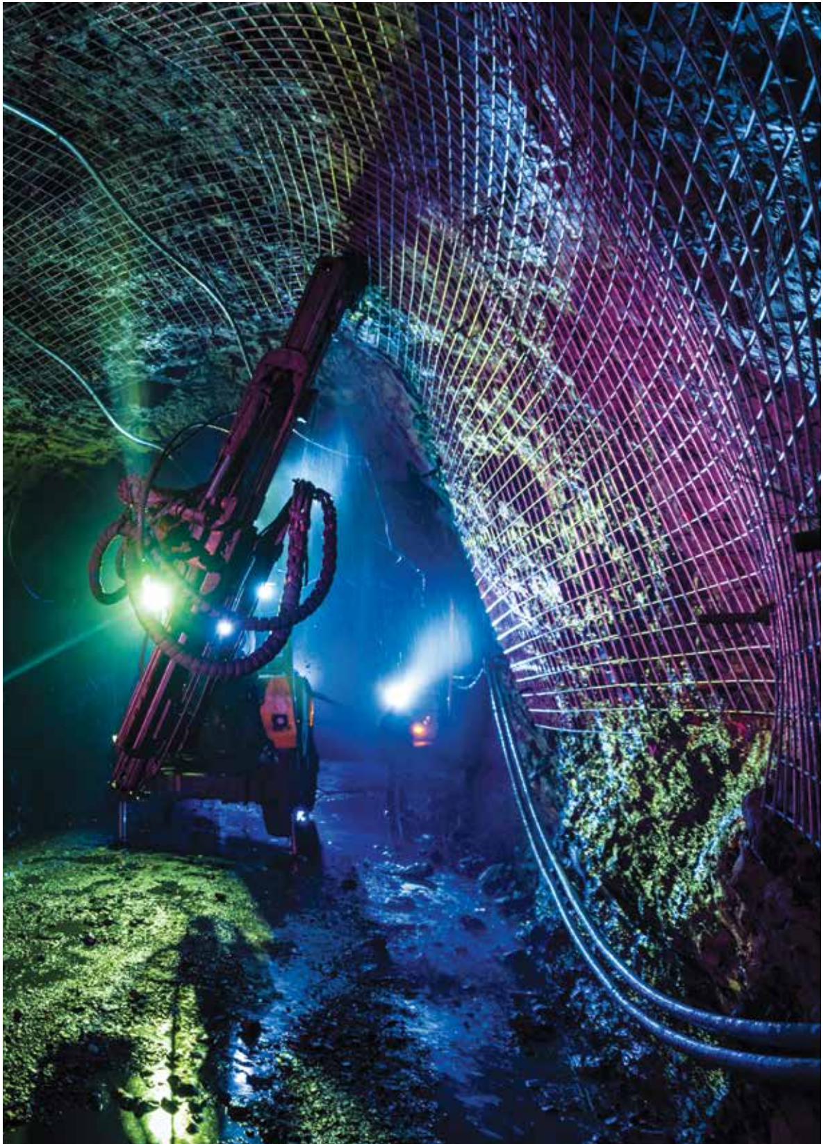
Inside view of Underground Zinc Mine
