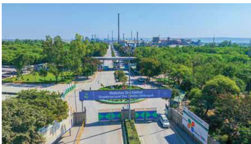
Chanderia Lead Zinc Smelter, HZL
