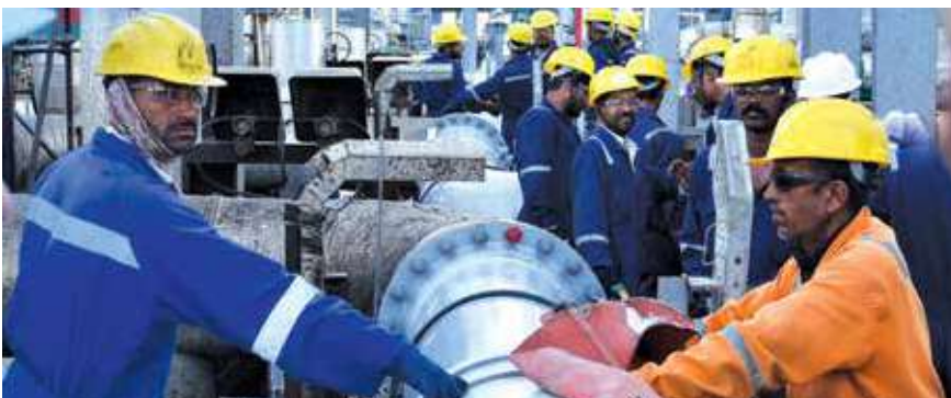
Shutdown maintenance activity at Cairn
