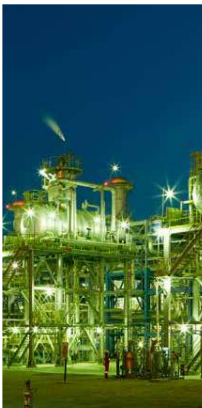
Mangala Processing Terminal at night, Barmer
