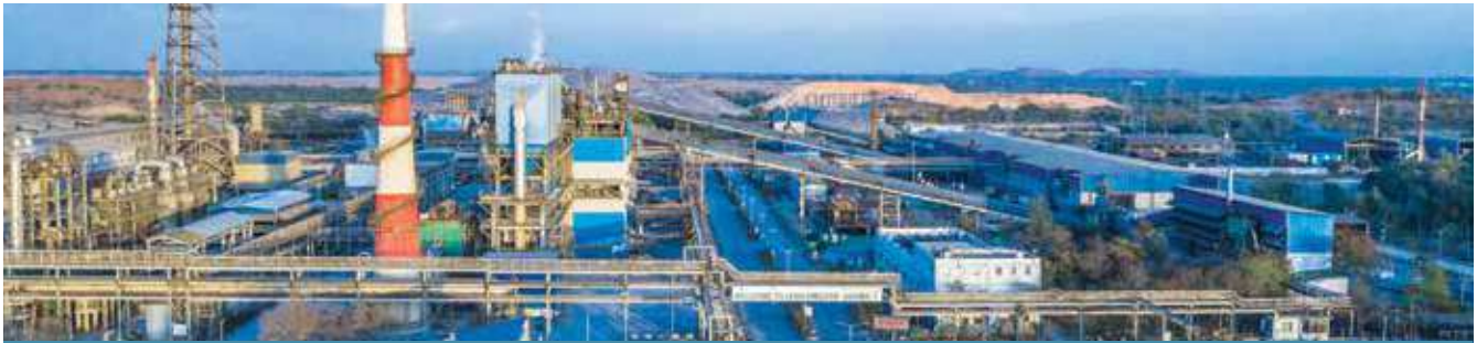
Dariba Lead Smelting Complex, HZL
