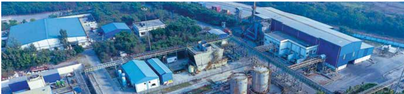
Aerial View of Pantnagar Metal Plant
