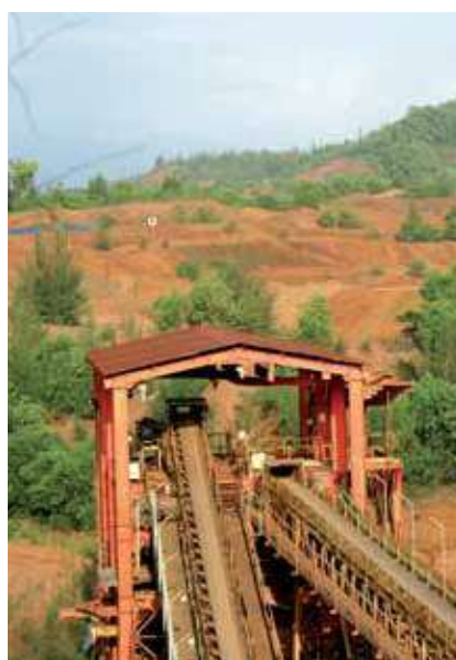
Processing Plant at Sesa Goa Mine
