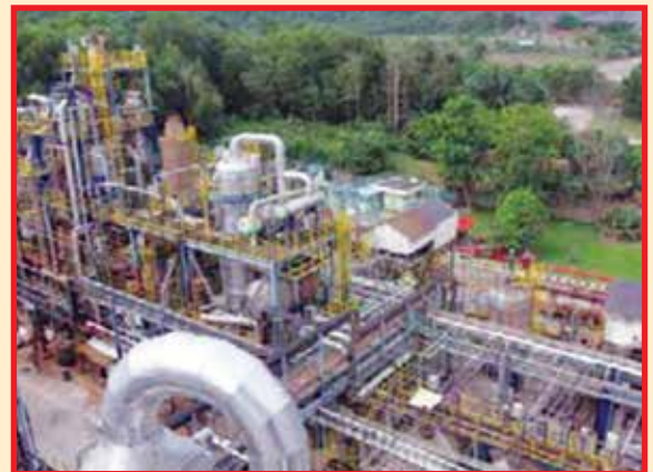
Maleic - Distillation Unit after Expansion : Malaysia
