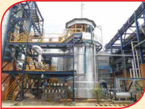
Revamp Project: A new Fired Heater - Utility Section
