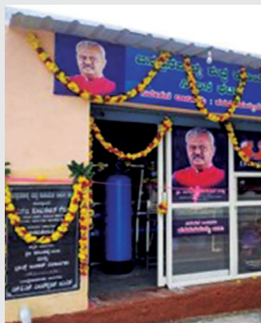
Constructed RO plants at villages
