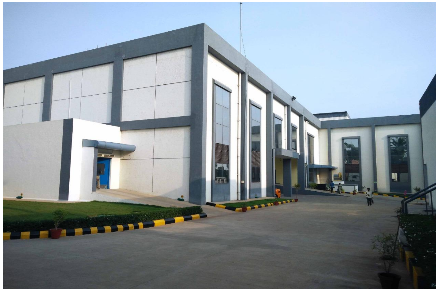
CP-I plant at Suthukeny, Puducherry
