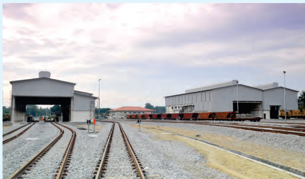
OLE PWay and Loco Workshops at Gemas Station, Malaysia
