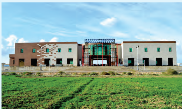
Relizane Station Building at Algeria
