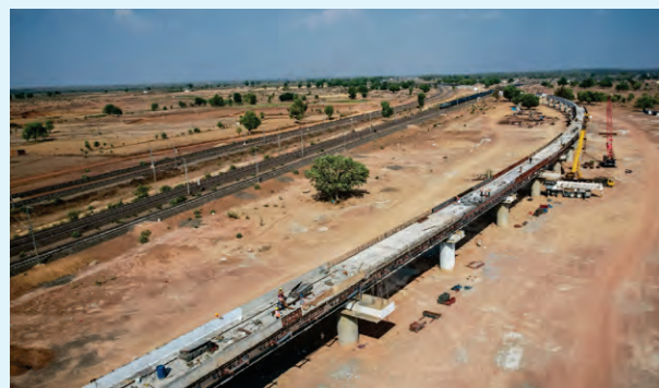
Katni Grade Separator Project
