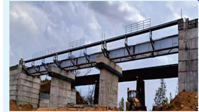
Composite Girder - Katni Singrauli Rail Doubling Project
