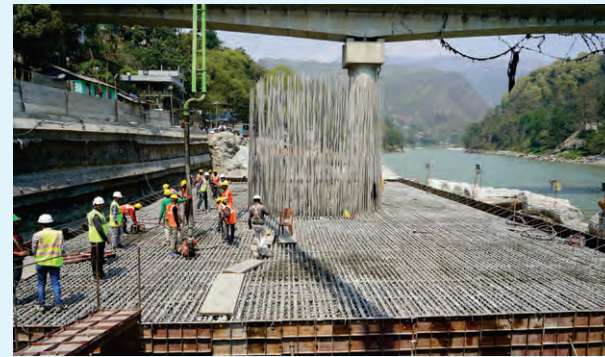
Bridge P P1 Pile Cap Casting in progress-Sivok Rangpo Railway Line Project
