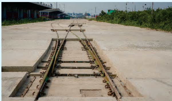
Ballast Less Track at Cargo Yard Mongla Bangladesh,
