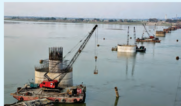
Well foundations in progress - Rampur Dumra Tal Rajendrapul Project
