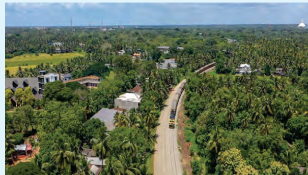
Completed track work between Anuradhapura-Omanthai, Sri Lanka
