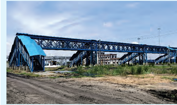
Nabinagar Super Thermal Power Project
