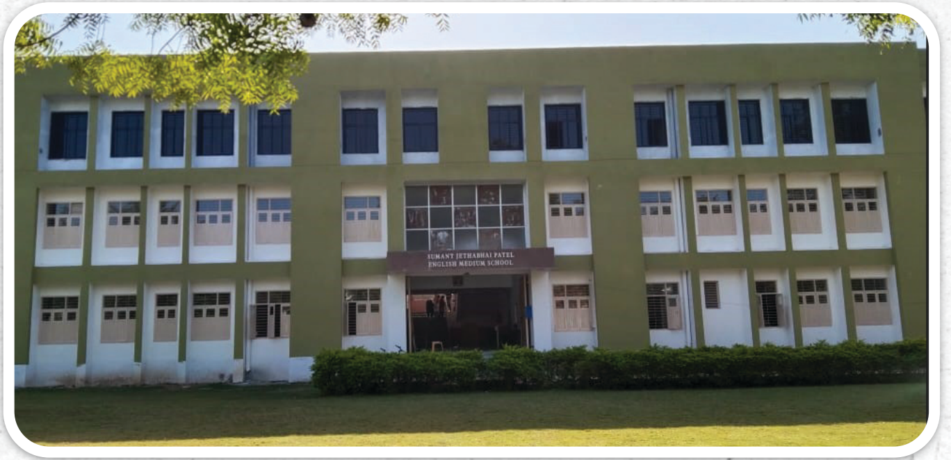
Completion of Construction of Second Floor at Sumant Jethabhai Patel English Medium School, Karamsad
