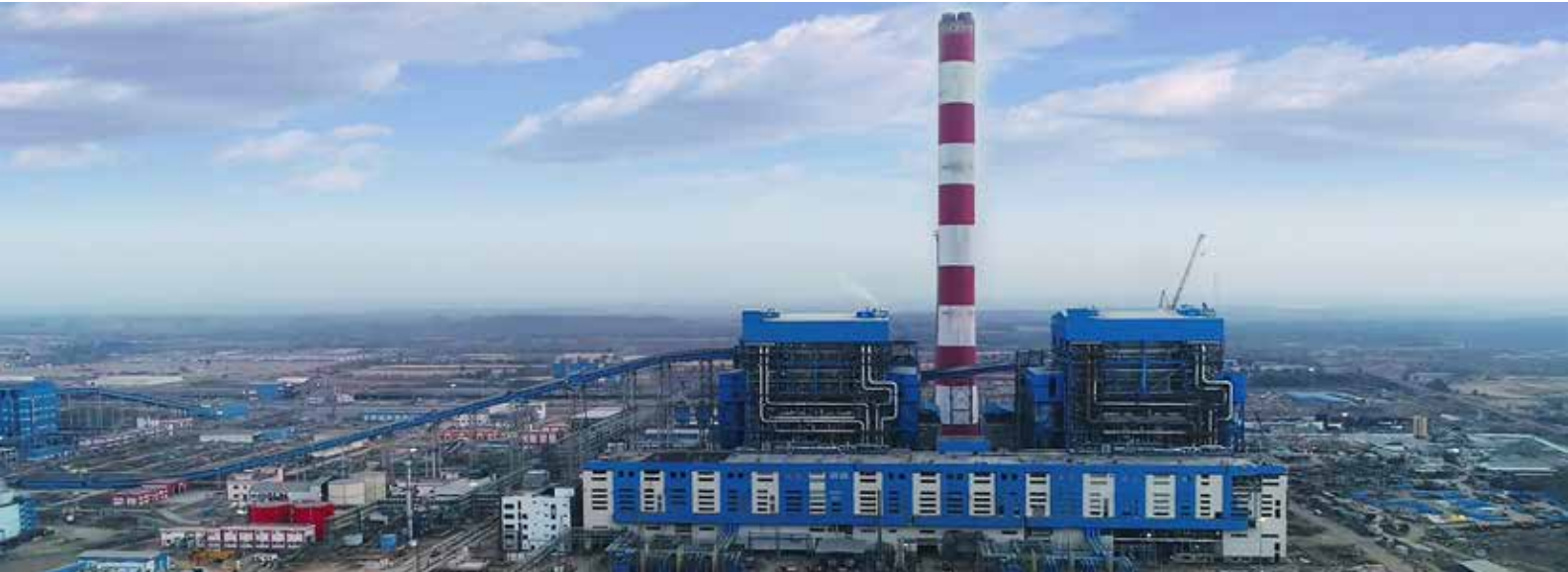
Flue Gas Desulphurisation (FGD) system at India's first ultra-supercritical thermal power plant, Khargone, Madhya Pradesh
