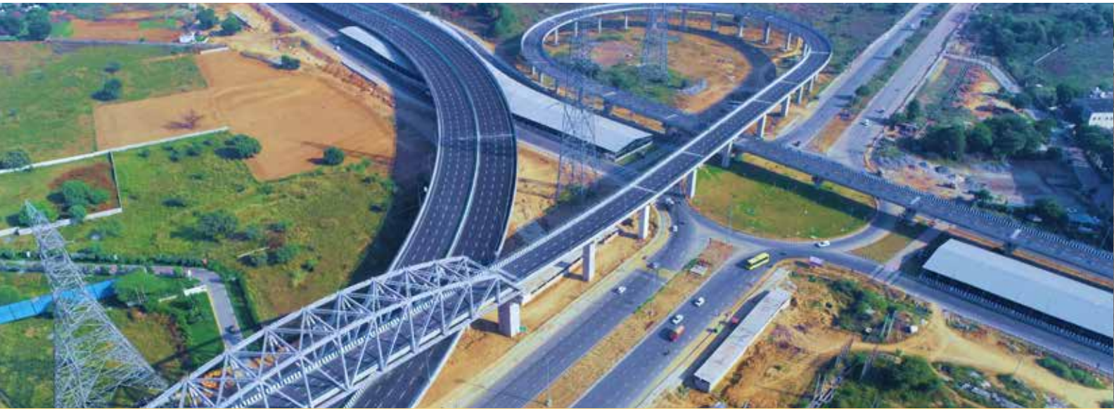
Dwarka Expressway, Haryana
