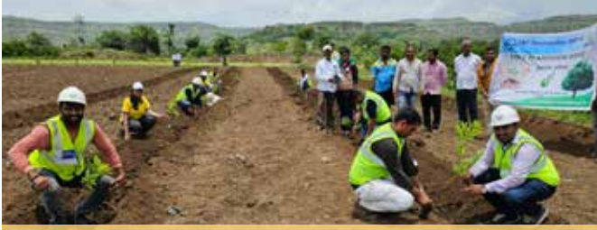
24x7 water project, Pune
