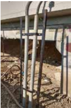
Support structure using steel scrap
