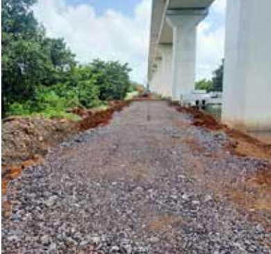
Approach road using steel slag
