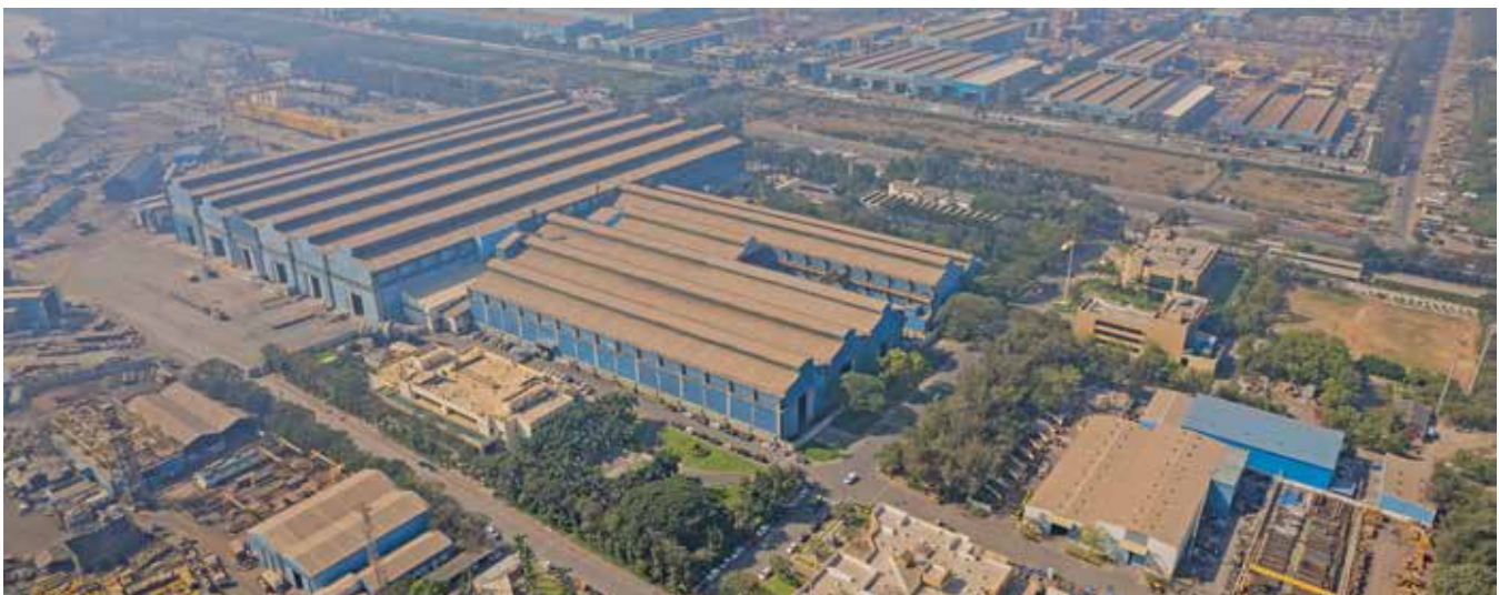
A. M. Naik Heavy Engineering Complex, Hazira, Gujarat
