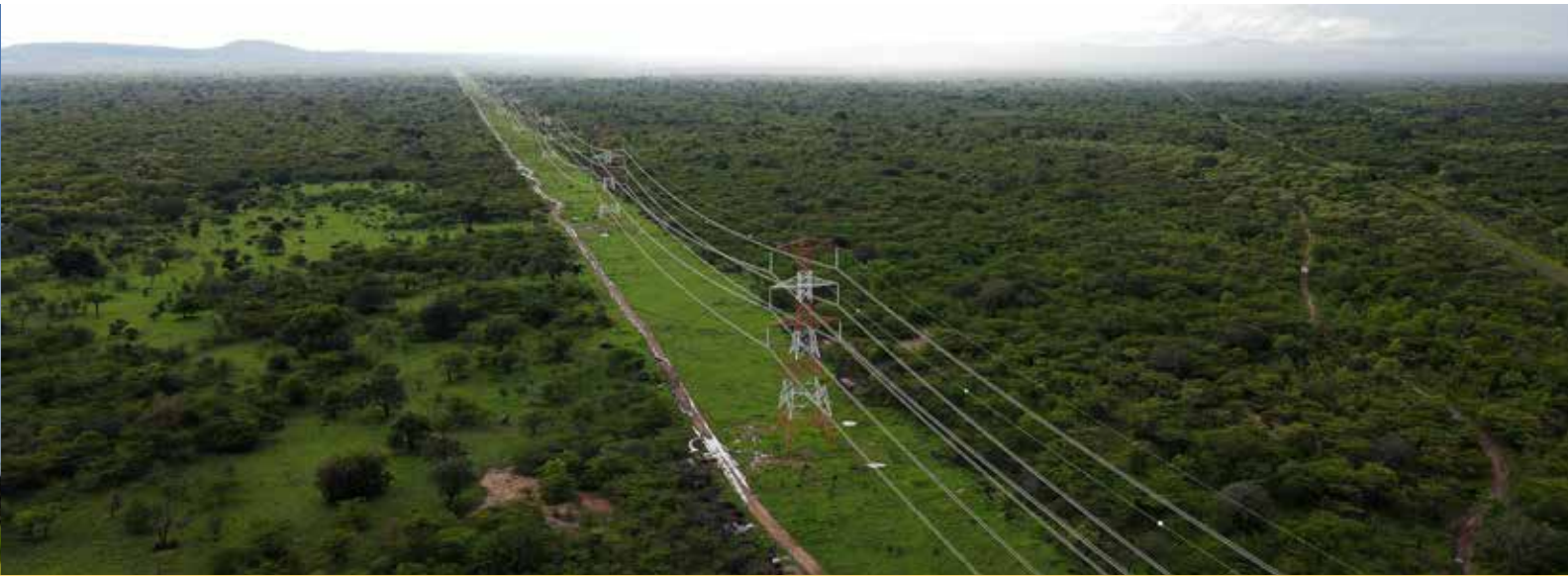
400kV JNHPP Chalinze Transmission Line, Tanzania
