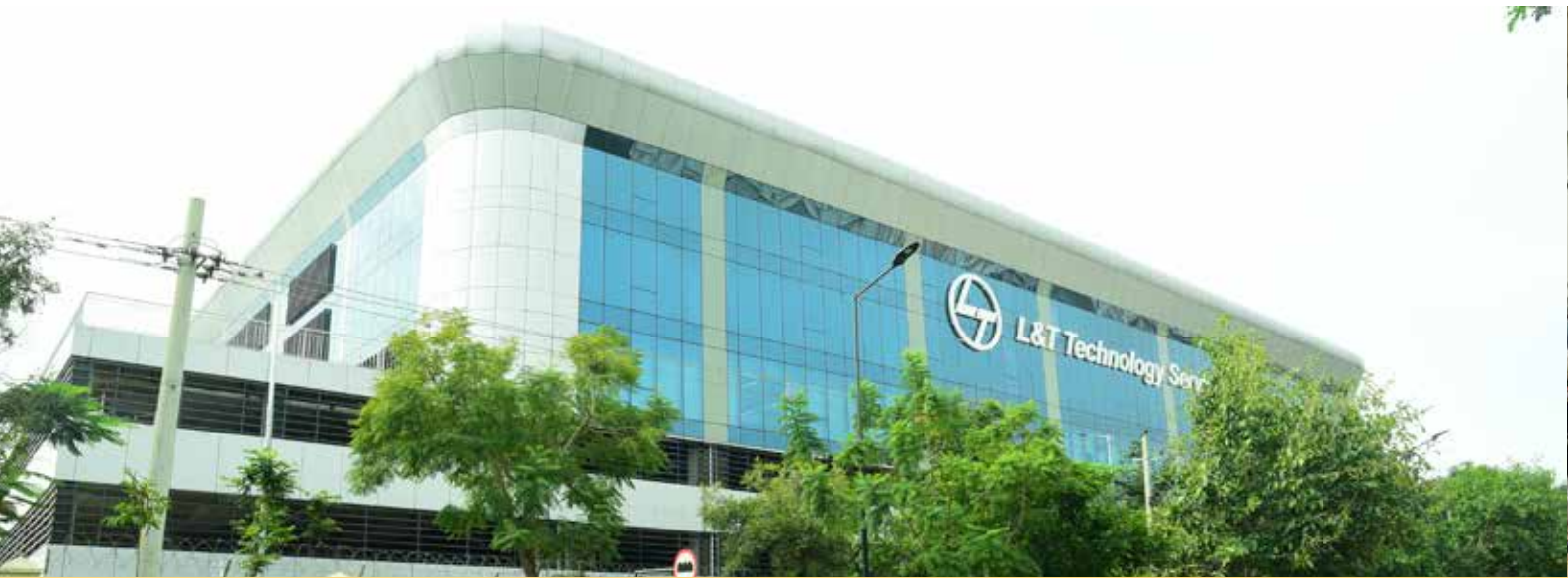
L&T Technology Services - Module X Design Centre, Mysuru, Karnataka
