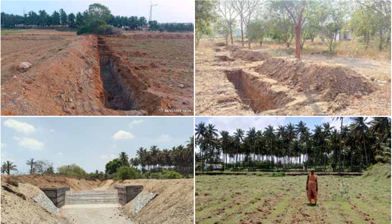
Water harvesting structures to enhance soil moisture content
