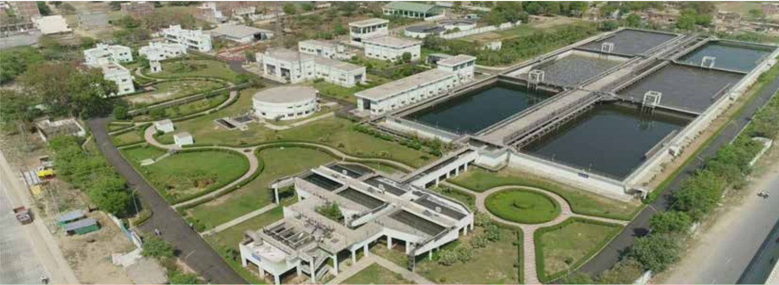
Varanasi Sewage Treatment Plant, Uttar Pradesh
