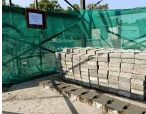
Paver Blocks from concrete waste
