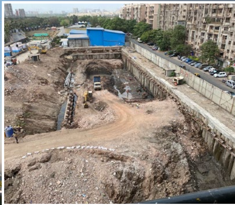
Piling Work Completed
