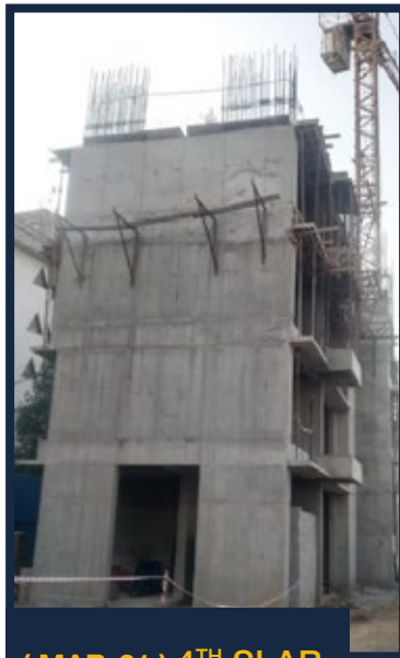
( MAR-21 ) 4 TH SLAB
