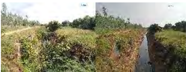
Noyyal Cannel After Cleaning Debris and Bushes
