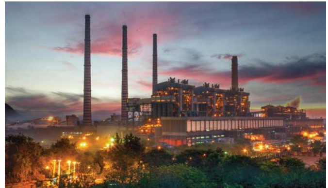
Korba-3 STPS (200 MW) equipped with BHEL-supplied sets achieved PLF of 97.7% and OA of 98.2%
