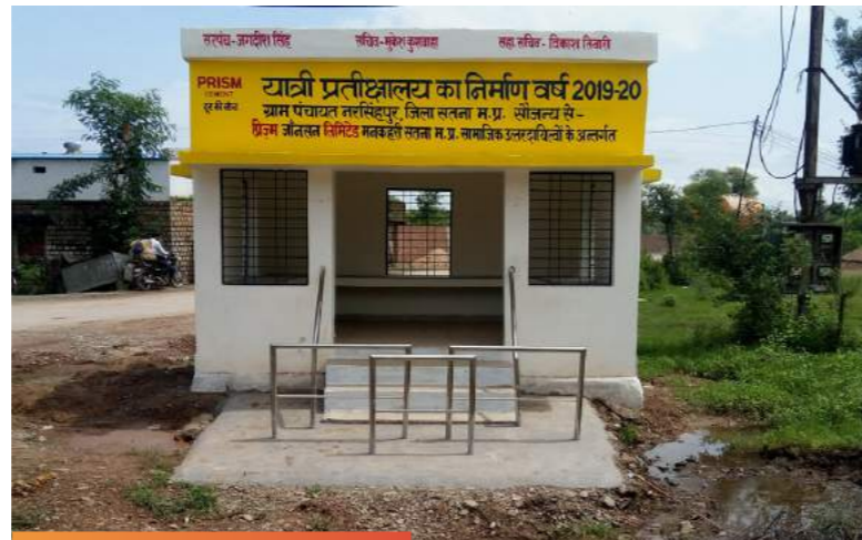
Construction of Bus Shelter at Kandaila Village
