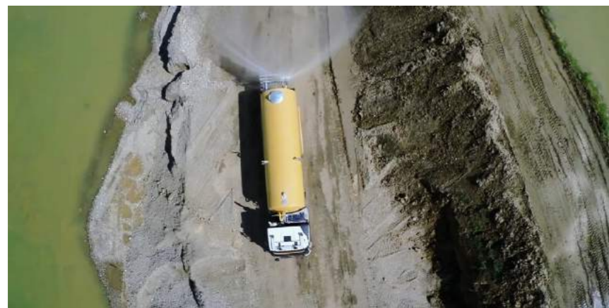
An automatic water fog canon used to suspend dust particles and reduce air pollution in dusty operational areas
