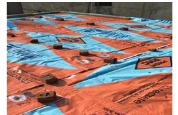
Prism RMC uses modular curing solutions as a water conservation measure saving up to 10,000 litres of water
