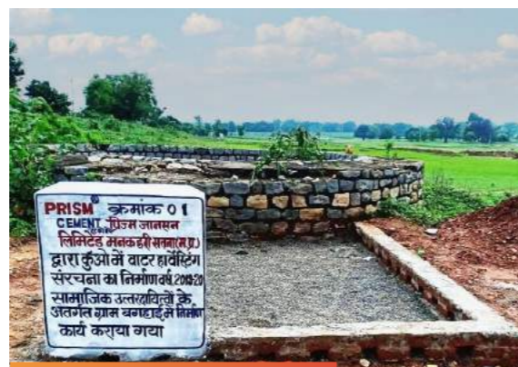
Construction of Dug Well Structure at Baghai
