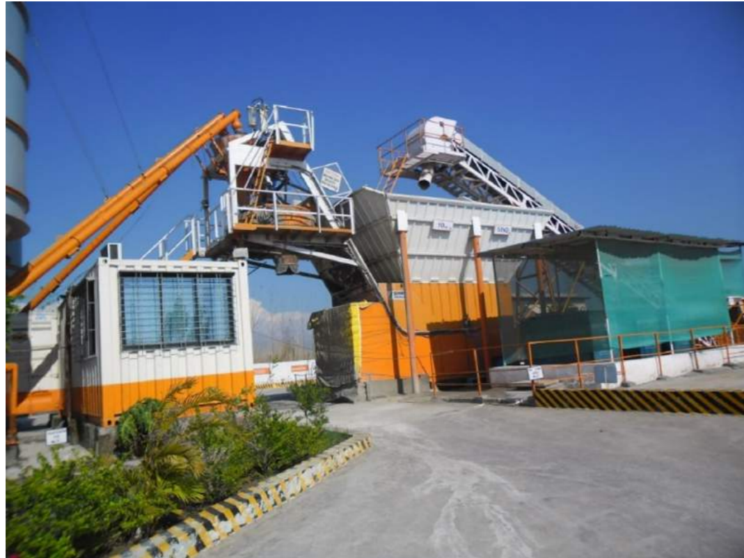
Machine guarding at one of our RMC plants
