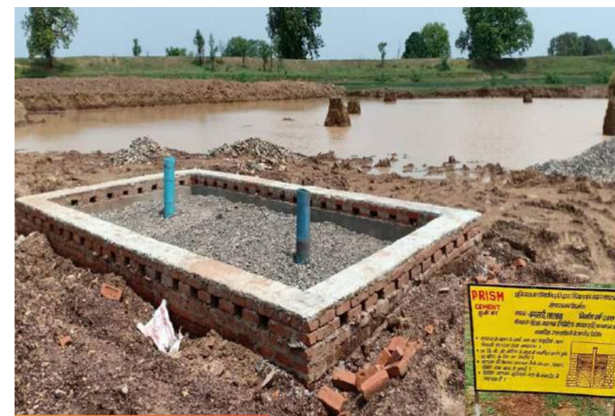
Construction of a double bore recharge shaft.
