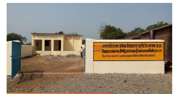
Construction of Boundary Wall at Chulhi School
