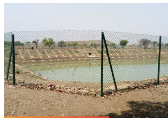
New Pond Excavation at Baghai Village
