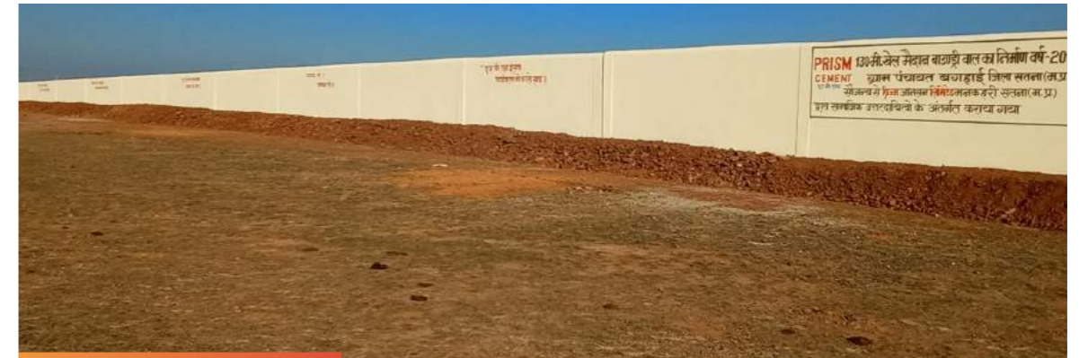
Construction of playground boundary wall at Baghai
