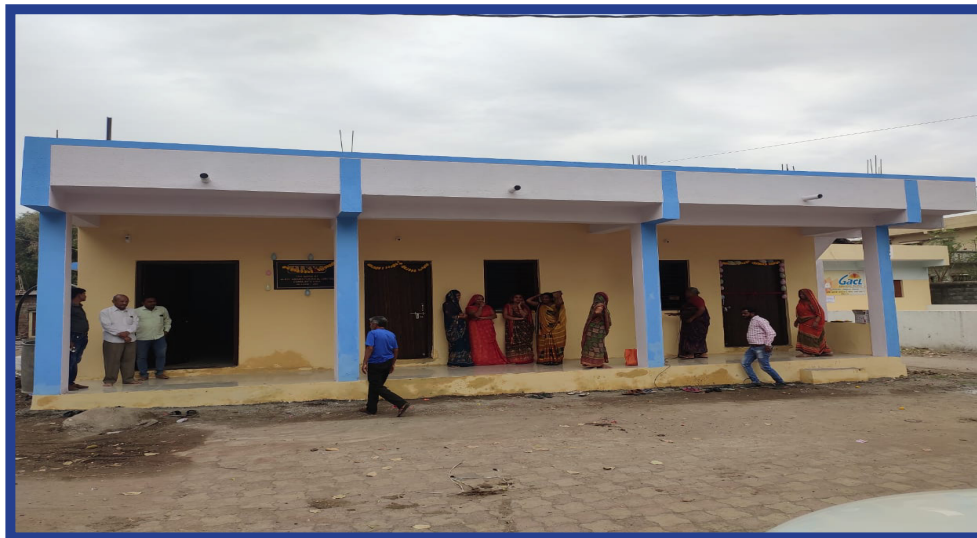
Construction of a Community hall at Vav Village, Dahej, Gujarat
