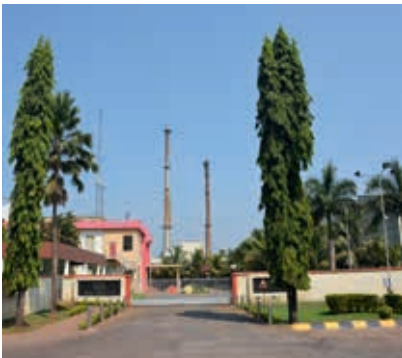
1997 manufacturing facility set up in Bicholim, Goa
