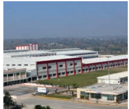
2012 manufacturing facility set up in Tahliwal, Himachal Pradesh
