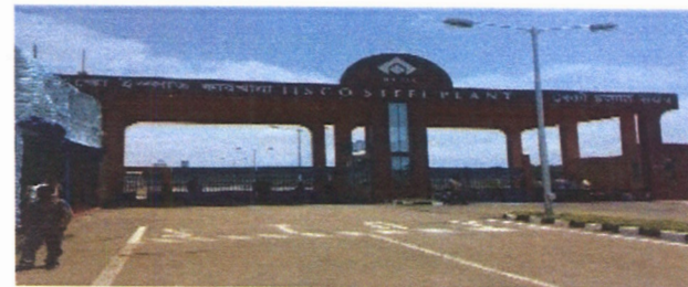
Approach Road 2 lane from GT Road at Neamatpur to Bumpur, West Bengal
