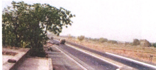
4 lane of km 41-51 of Agra Dholpur of NH-46 (earlier NH 3), in the state of Rajasthan
