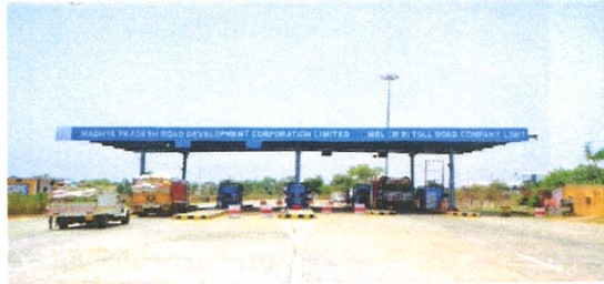
Strengthening, Widening, Maintaining and Operating 18.303 kms Waraseoni-Lalbarra Road in the state of Madhya Pradesh
