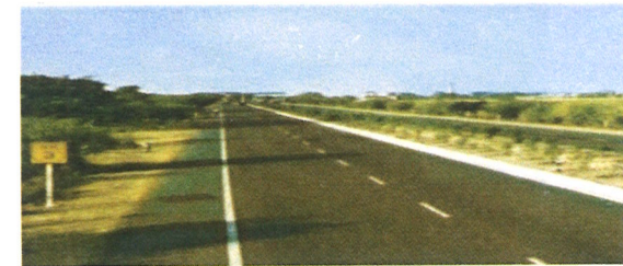
4 laning at Agra- Gwalior section, NH-2, in the State of Madhya Pradesh
