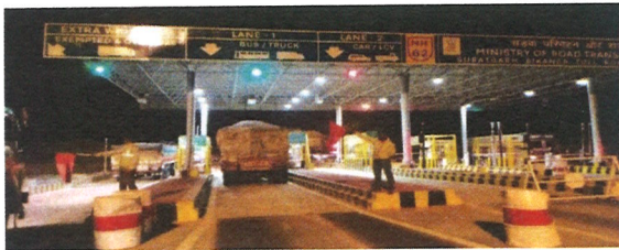
Development & Operation of Bikaner- Suratgarh Section of NH-62 (earlier NH-15) in the state of Rajasthan
