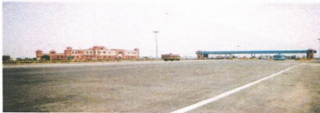
Toll Plaza construction at Delhi –Agra, NH-44 (earlier NH-2)
