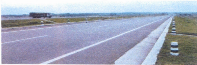
Maintenance of NH-19, (earlier NH-2) Barwa Adda –Panagarh Section (KM 398.75 –KM 512.00) in the state of Jharkhand & WestBengal
