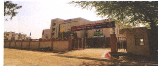
Construction of Police station & Residential Quarters, Hari Nagar, Delhi for MHA, Delhi Police through RITES Ltd.
