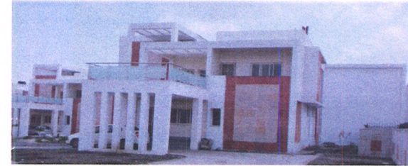
Construction of Director, Dean Bungalow, QIP Centre & Accommodation for School of Planning & Architecture at Bhopal
