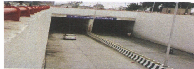
Construction of RUB at Badli, New Delhi
