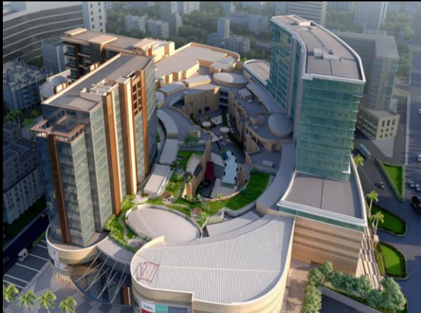
Phoenix MarketCity + Fountainhead Office Towers, Pune
