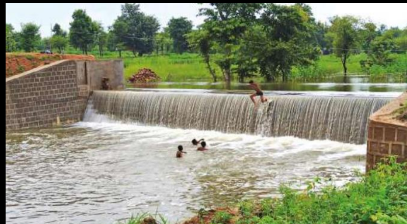
Recharging Ground Water Table
