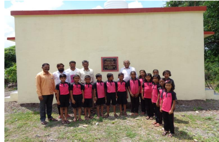
Constructed Ladies And Gents Toilet Block At Innovative School Ankoli Taluka Mohol District Solapur Dt 03.09.2022
