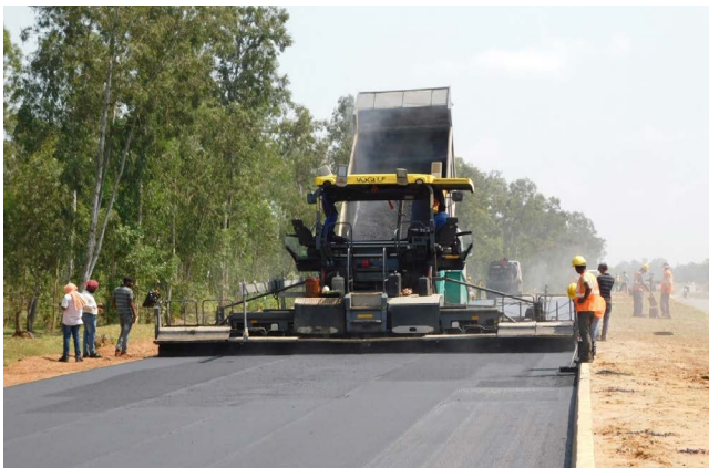
● Upgradation of Baharaghora-Singhara Highway in Odisha
