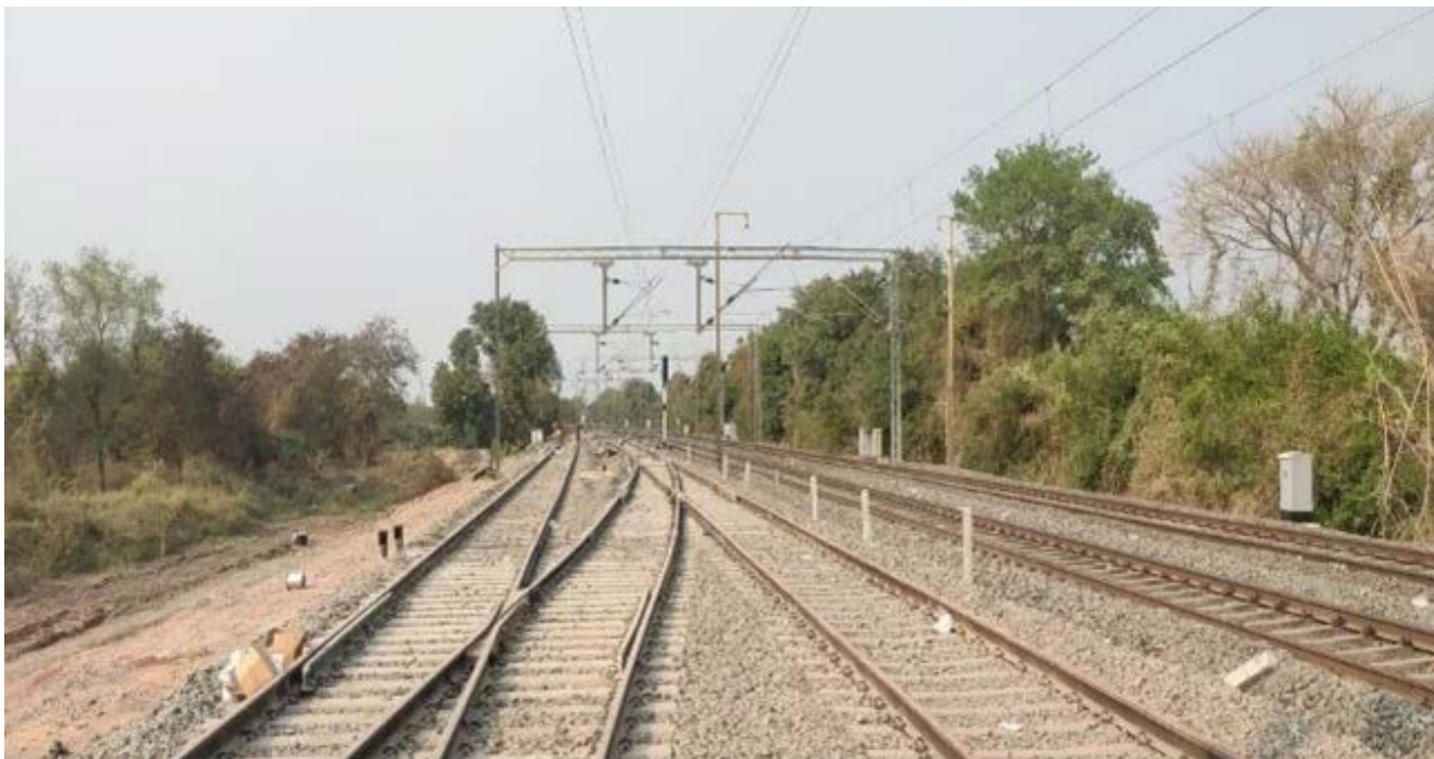
● Laying of crossover in main line at Varnama.
