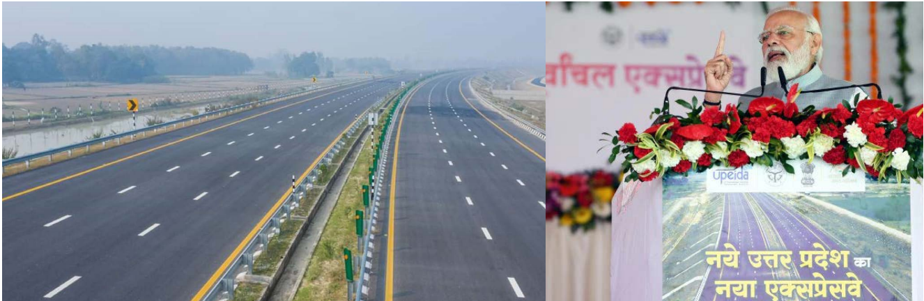
● Hon'ble Prime Minister Mr. Narendra Modi at the inauguration of Purvanchal Expressway, for which RITES was construction supervisor-cum-ETA
