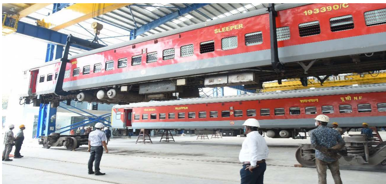
● Setting up of facilities for refurbishment of LHB coaches at New Bongaigaon.
