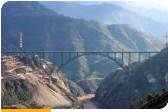
Railway bridges & girders
