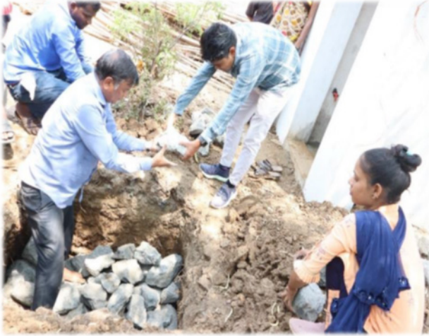
Construction of Soak pit in Doadwada
