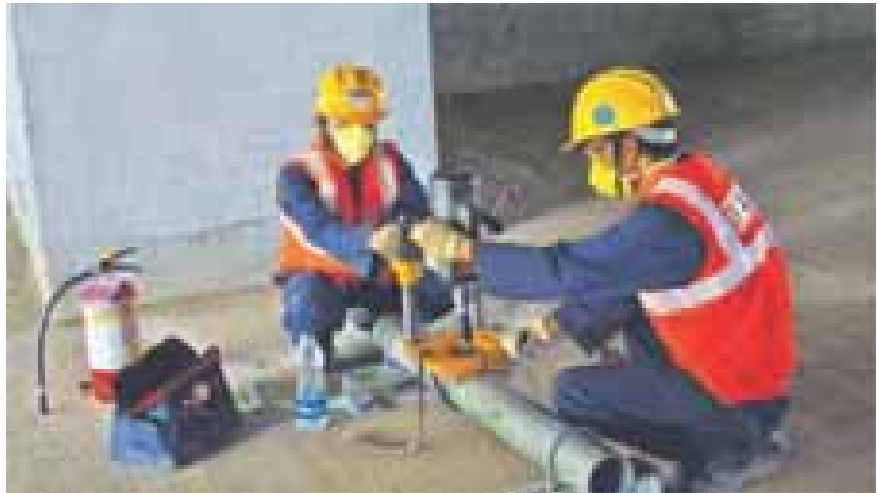
Safety practices being adhered to at a project site
