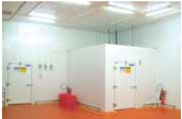
Cold Room installation for Domino's, Kolkata
