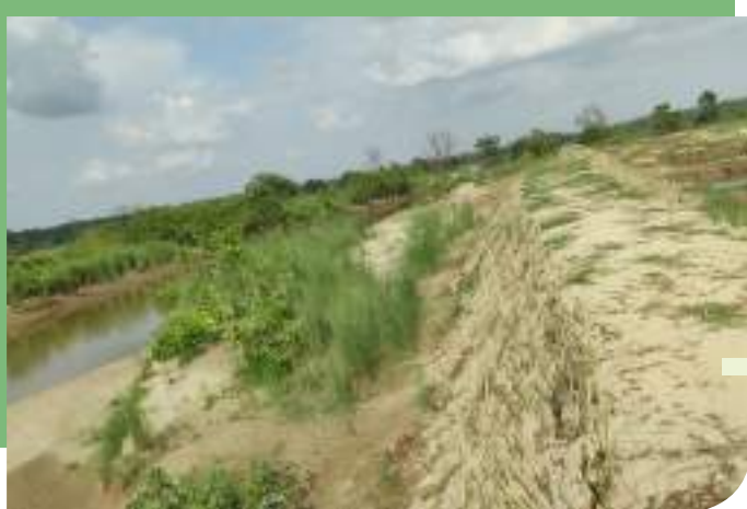
Village Mankapur block- Palia 2700 mtrs bund formation and repair work
