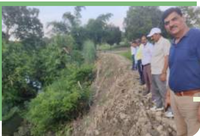
Village Gola-block Palia 90 mtrs bund repair work
