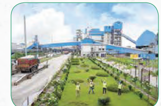
Panagarh Cement Plant
