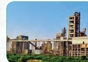
Nimbol Cement Plant
