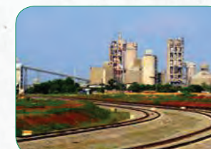
Sonadih Cement Plant
