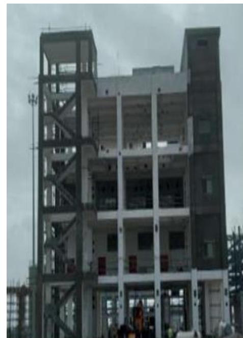
High pressure, multi-purpose fluorination plant
