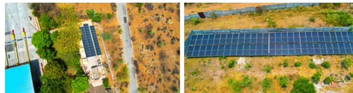
Rooftop installation at Bassi Toll Plaza
