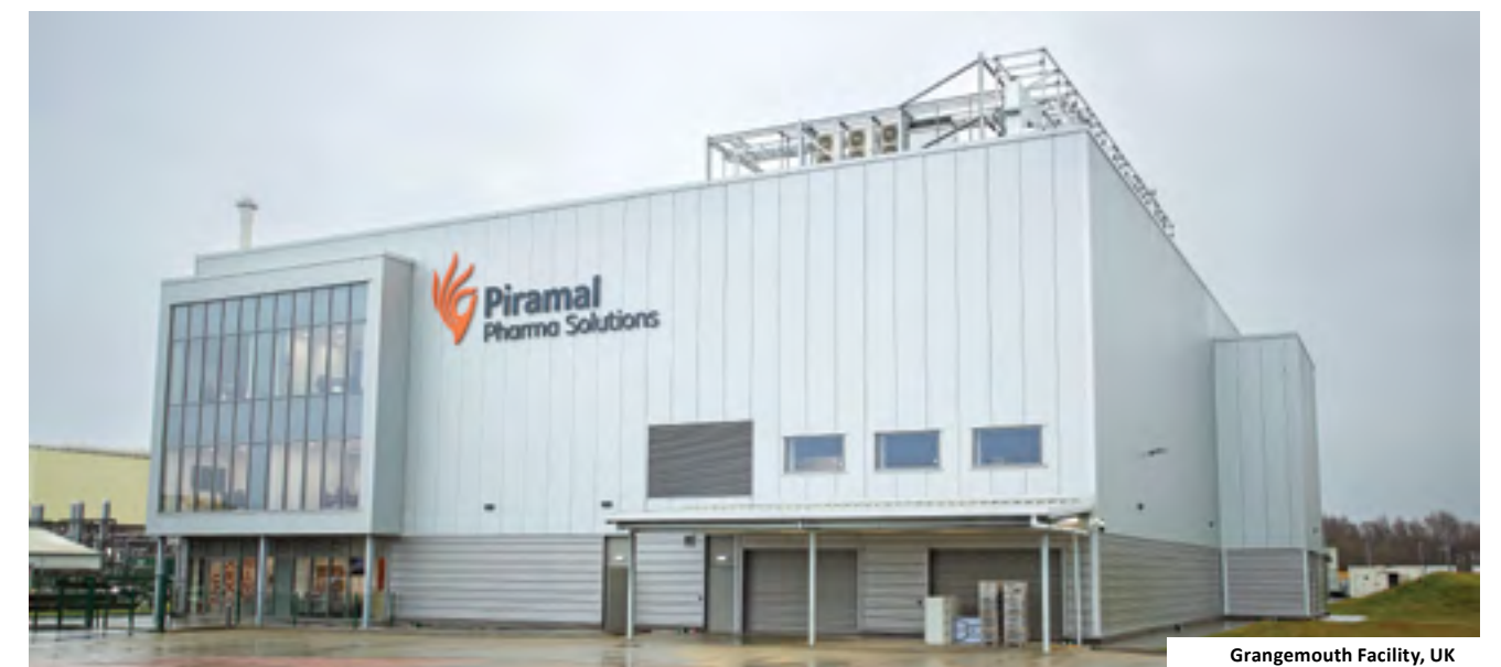
Grangemouth Facility, UK
