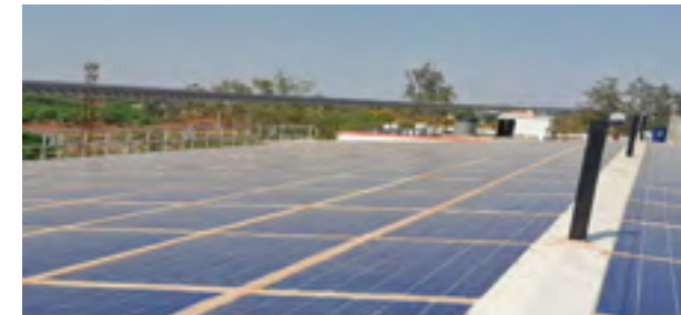
Solar panel installation at one of our sites
