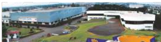
Menon Bearings plant at Kolhapur,
