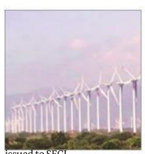
issued to SECI. Although the company, in its petition to the CERC, has not specified the project for which it wants to cancel the PPA, industry sources said the matter pertained to the 100 MW wind farm Sprng was to build in Dhar district of Madhya Pradesh. The company was issued the letter of award for the project in
