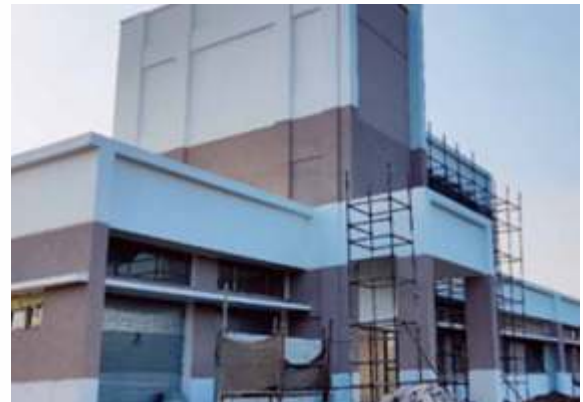
DFC Station Building at Ancheli (Gujarat).
