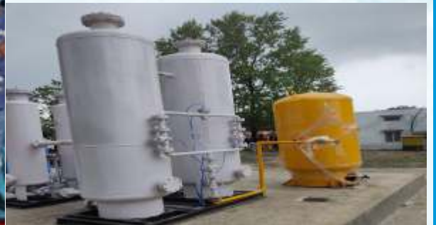
Installation of Oxygen Generating Plant at Divisional Railway Hospital, Samastipur, District of Bihar
