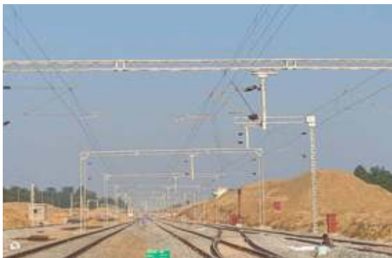
CERL – I Electrification Work
