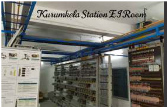
CERL – I Electrification Work
