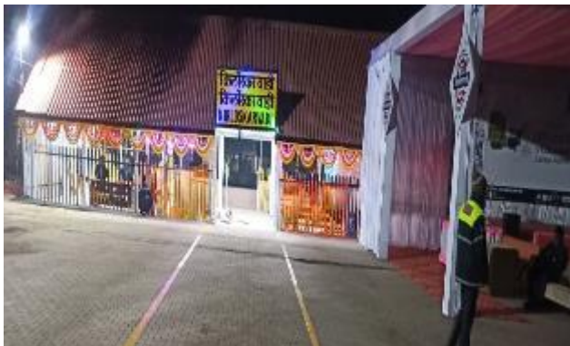
Renovation of Kirloskarvadi Station
