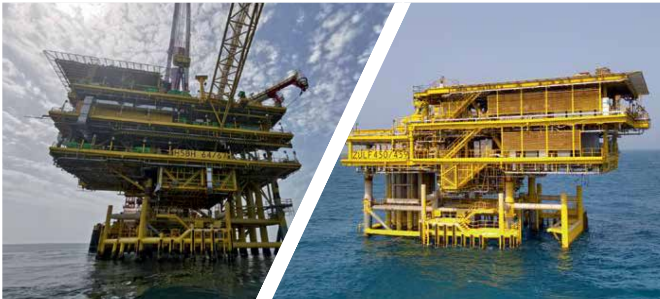
One of the Three Gas PDMs installed in Hasbah Field, Saudi Arabia
