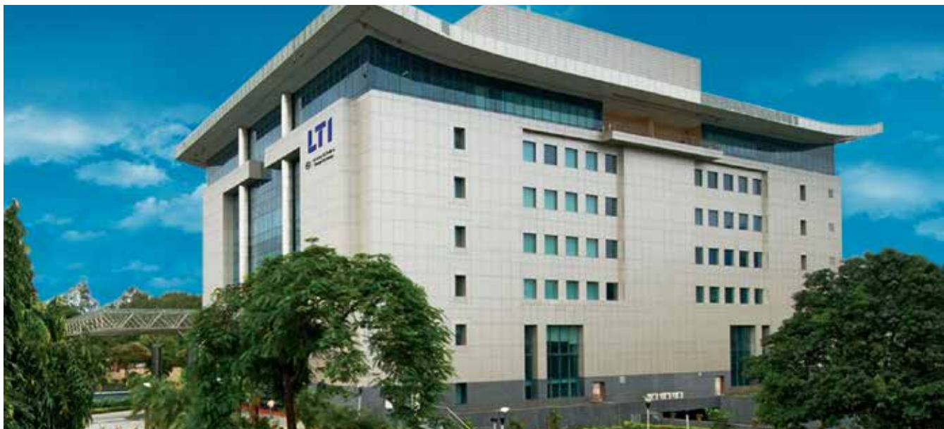
LTI Headquarters, Powai, Mumbai
