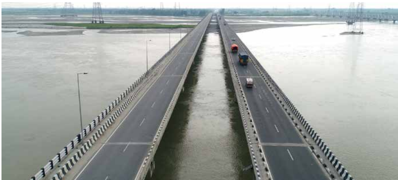
Ghoshpukur Salsalabari Road Project
