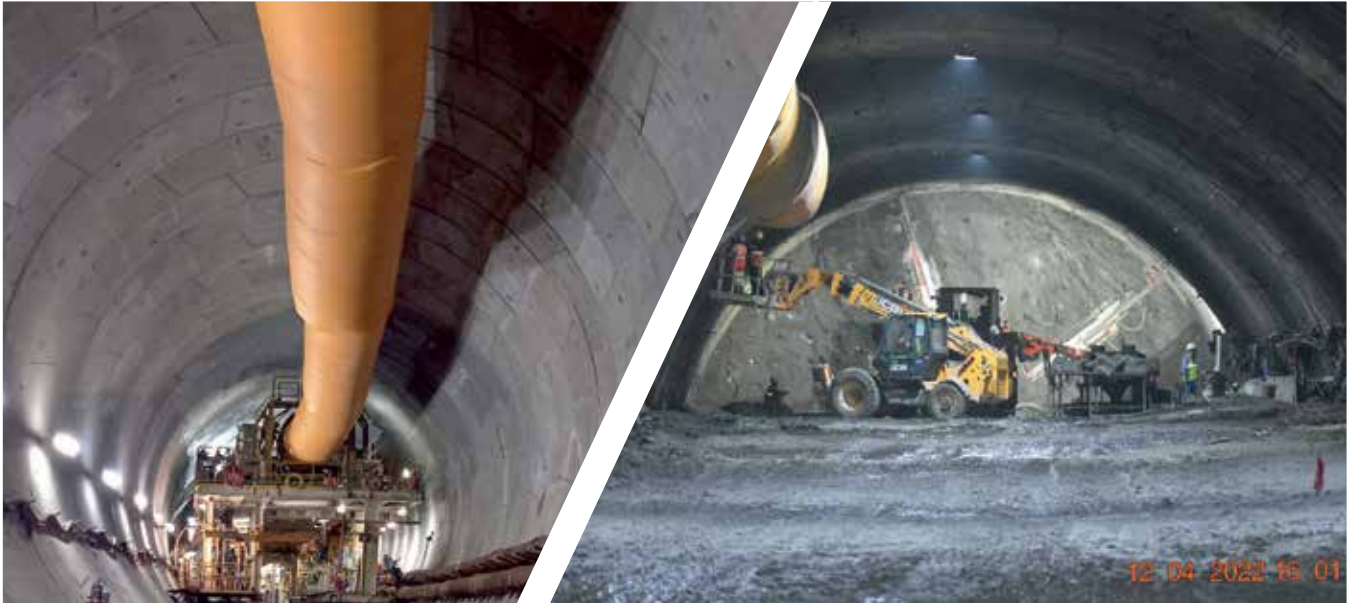
Bangalore Metro – an underground section
