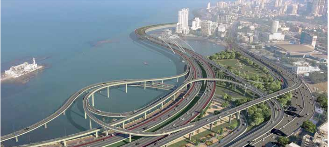
The Mumbai Coastal Road Project. L&T is executing Packages 1 and 4.
