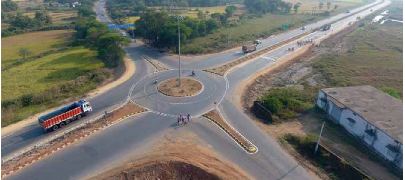
Major junction at Sambalpur-Rourkela Tollway Limited
