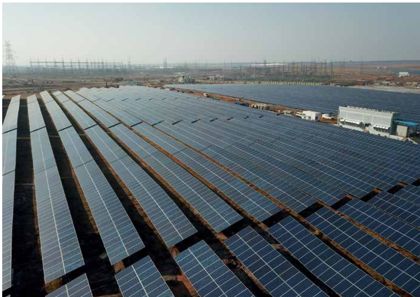
250MW Solar power plant at Rewa. Madhya Pradesh
