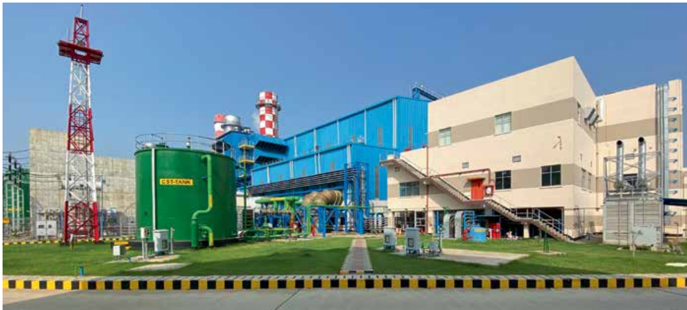
400 MW Bibiyana South Combined Cycle Power Plant, Bangladesh
