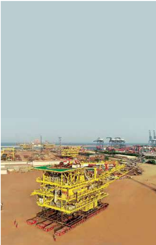
Gas Production Modules fabricated at LTHE's Oman Facility for Hasbah II
