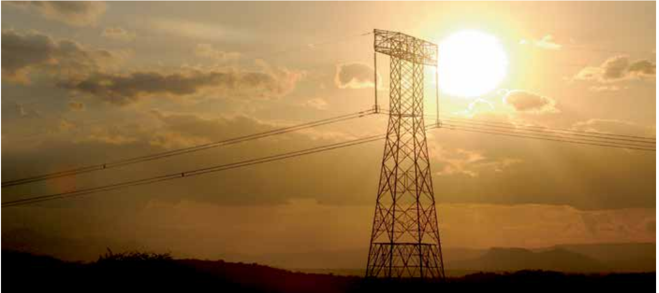
500 kV HVDC Transmission Line, Kenya
