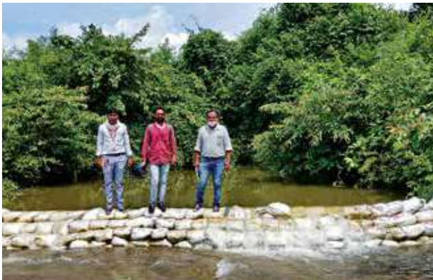
Boribandh is a low cost water harvesting structures used for the harvesting of rain water. 3,960 boribandhs have been constructed.
