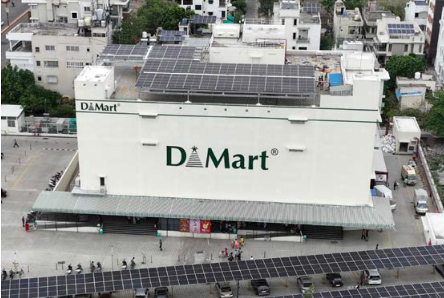
Rooftop Solar Panels and Carports
