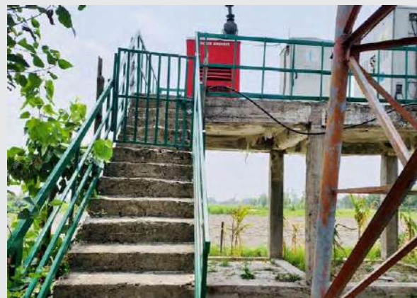
Infrastructure elevated to combat flood impact
