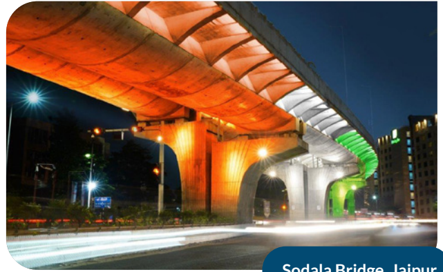
Sodala Bridge, Jaipur
