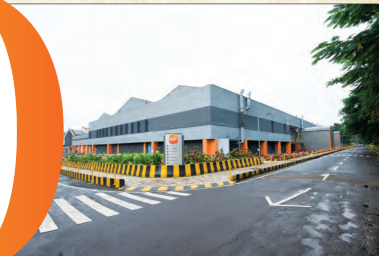
▲ GSK India's present-day manufacturing factory located in Nashik, Maharashtra
