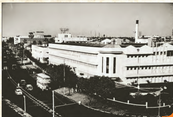
▲ Glaxo's first factory at Worli, Bombay (now Mumbai), Maharashtra
