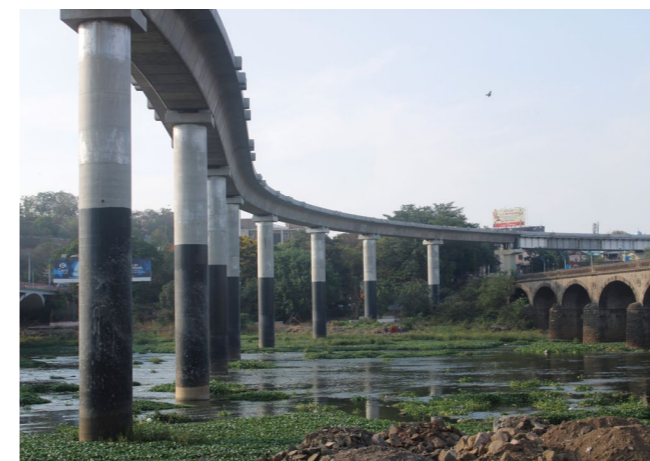
● Pune Elevated Metro
