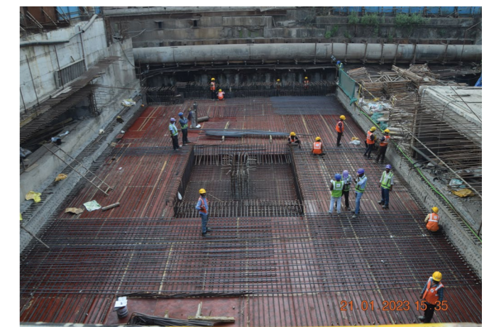
● Mumbai Metro Line 3
