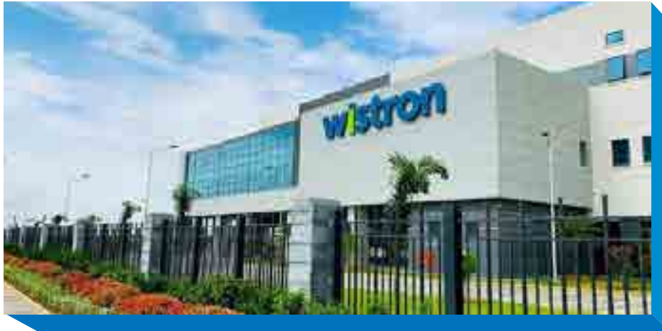
Mechanical, Electrical and Plumbing (MEP) works for Wistron Infocomm's factory expansion project, Bengaluru
