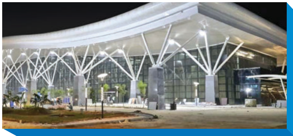
Glimpse of the upcoming Sir M. Visvesvaraya Terminal in Bengaluru, which is the first centrally air-conditioned terminal in India, where Blue Star has supplied oil free centrifugal chillers
