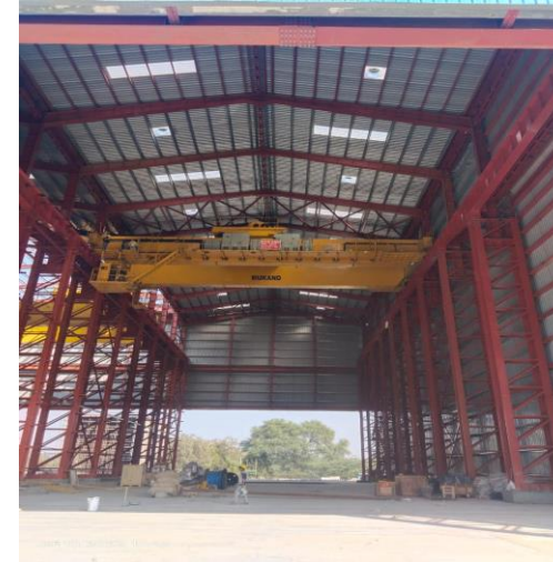
Inside working area with crane installed
