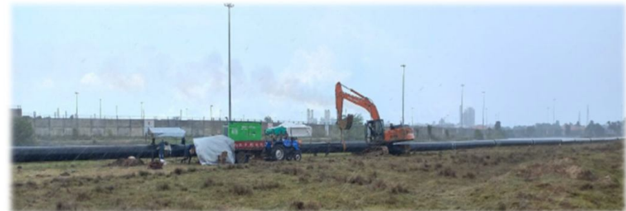
Setting up slurry pipeline
