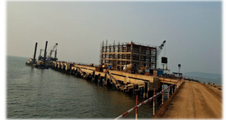
LPG construction at Jaigarh Port
