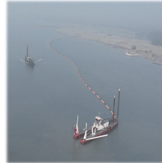
Dredging work underway at Jatadhar
