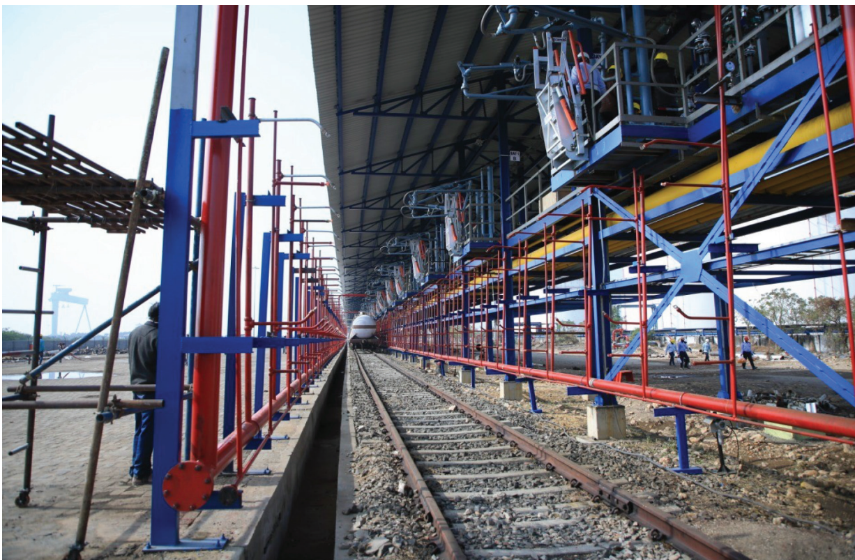
First LPG loaded rake departing Pipavav Terminal
