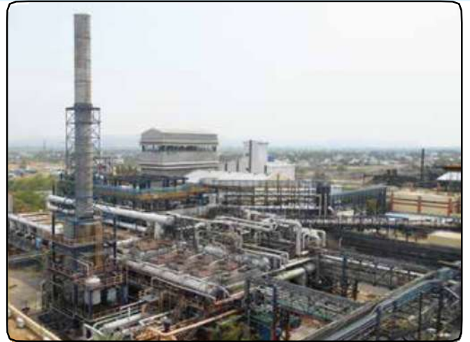
PA Plant - Ranipet, during revamp
