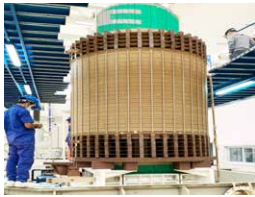
Dhule ICT Repair work
